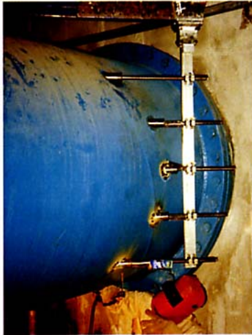
Welding saddles and connecting stop-cocks
